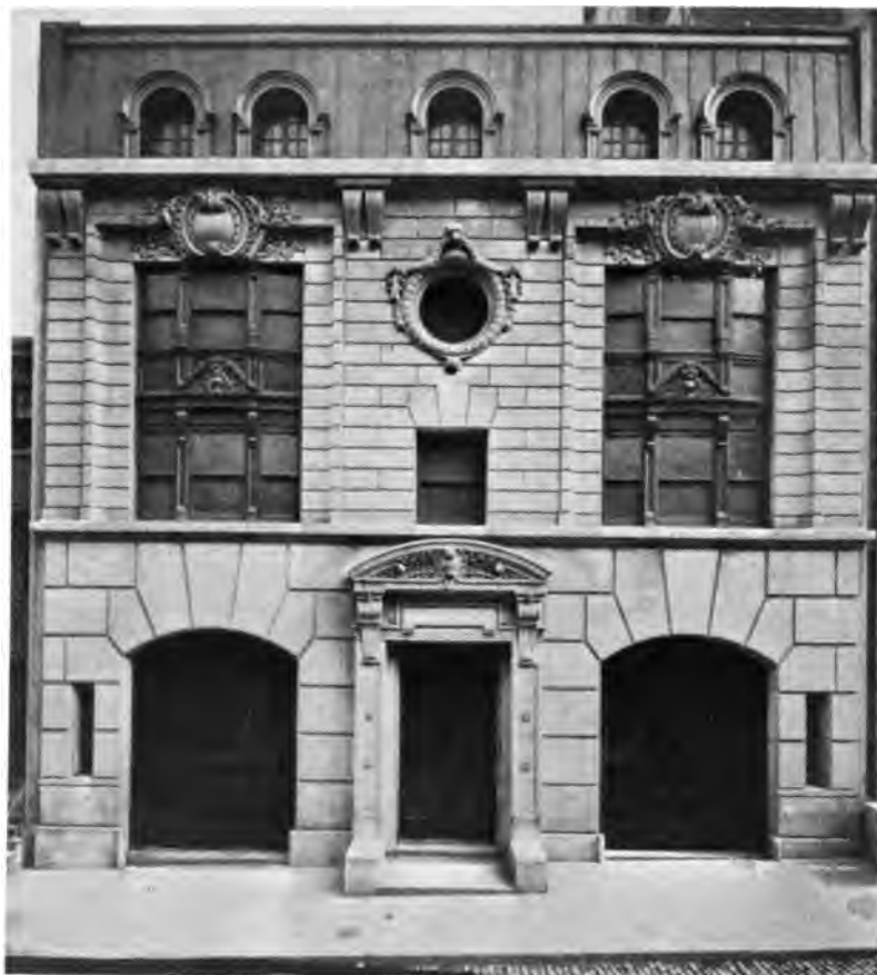
EXTERIOR OF SUB-STATION NO. 11
